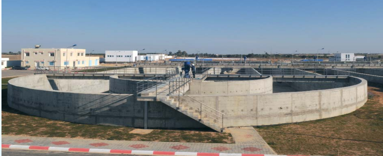
Station d'épuration de Kairouan II Kairouan II Wastewater Treatment Plant
