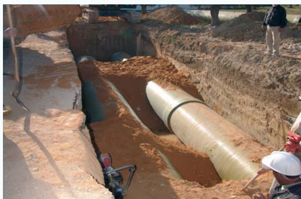
Pose de tuyaux en PRV Fiber glass pipe laying works
