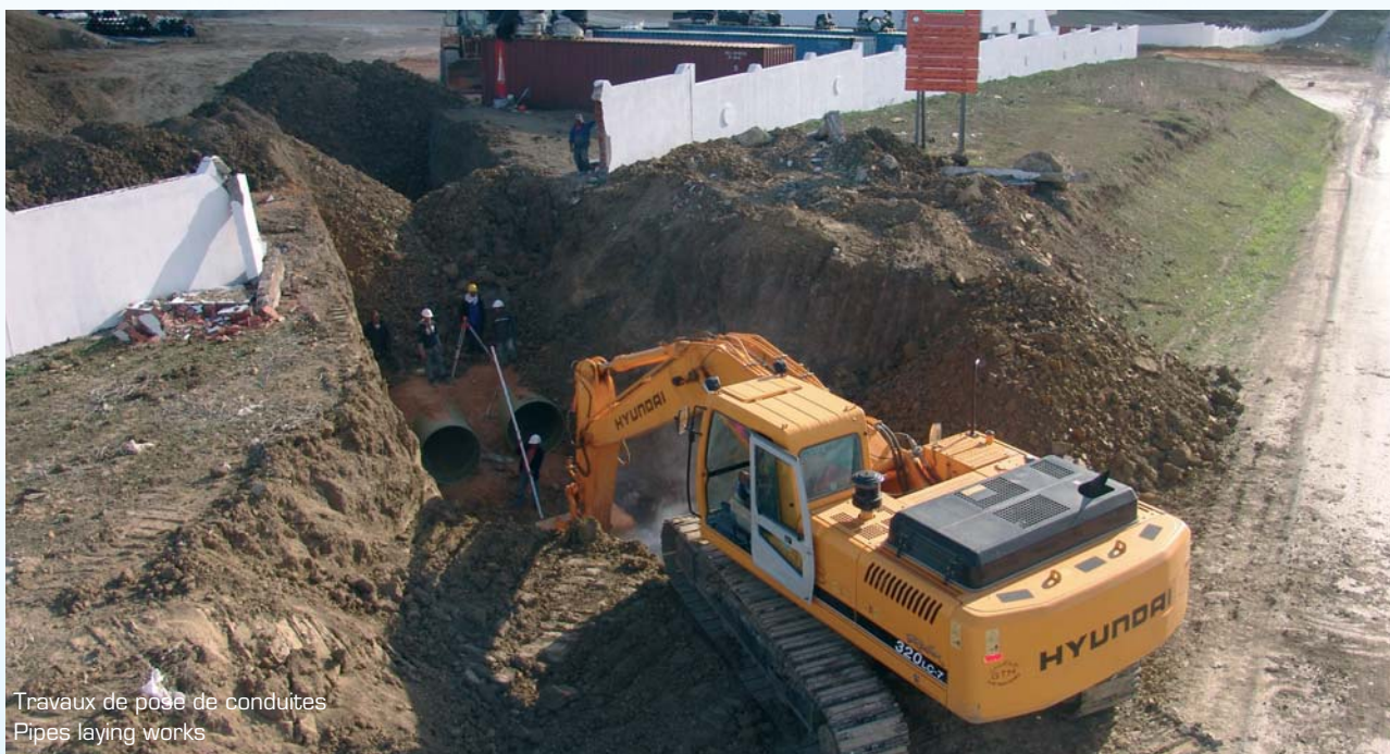
Pose de tuyaux en PRV Fiber glass pipe laying works
