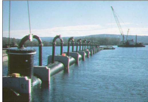
An **ALTERNATING MULTI-PORT** diffuser for **MUNICIPAL WASTEWATER** discharge into a **LAKE** under construction (Photo: G. Jirka).
